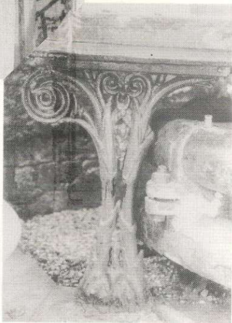
Figure 21 (right). Detail of a cast iron stanchion holding the plant shelf in the central palm house, Curvilinear Range, National Botanic Gardens, Dublin.
