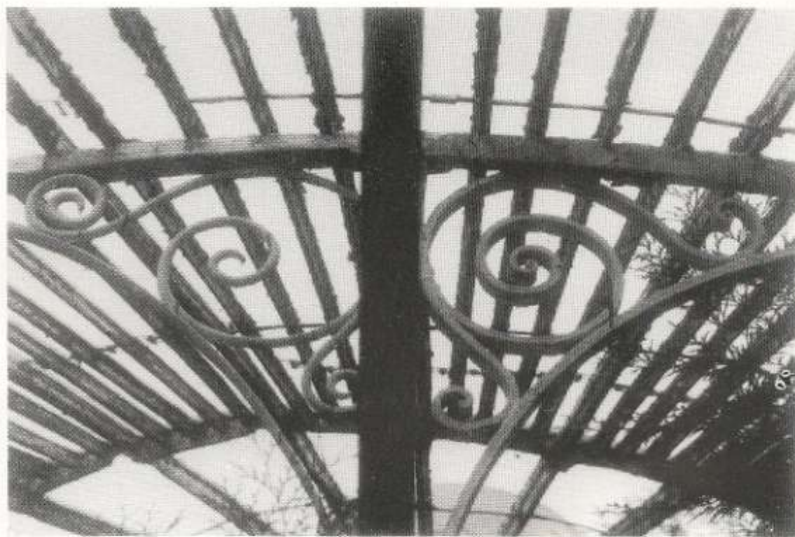
Figure 26. Detail of the junction of the old roof with the new roof added in 1868-9, east wing of the Curvilinear Range, National Botanic Gardens, Dublin. Note the differences in the scrolls.
