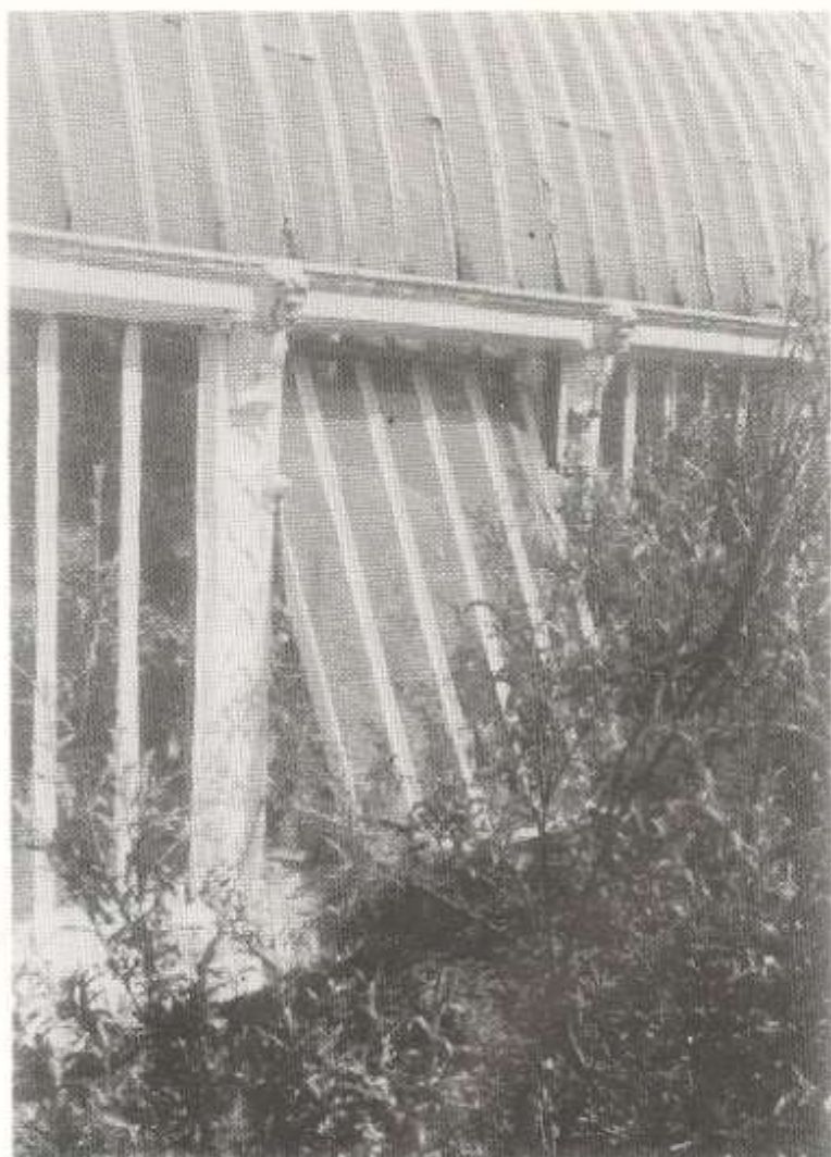
Figure 11 (right). Detail of a swivelling sash of the east wing of the Curvilinear Range, National Botanic Gardens, Dublin.
