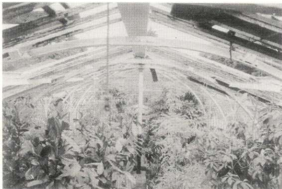
Figure 25. Interior of the west wing showing the span roof supported by the butterfly trusses, Curvilinear Range, National Botanic Gardens, Dublin.
